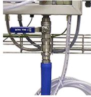
4. ▶ Open the valve under the Foamatic satellite.
