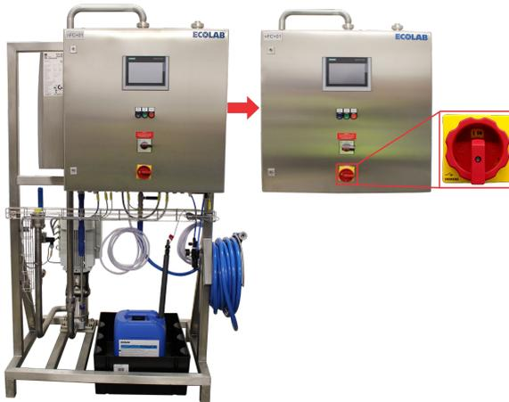
The EMERGENCY STOP switch is on the door of the control panel right under the UPS switch.
